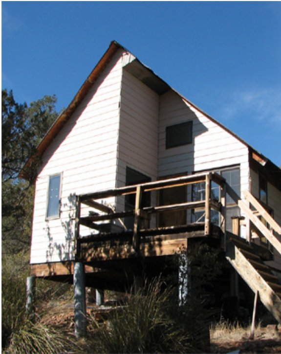
Renovated winter cabin
